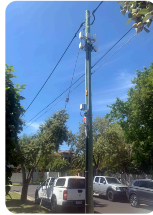
Example 5G small cells installed on street poles
