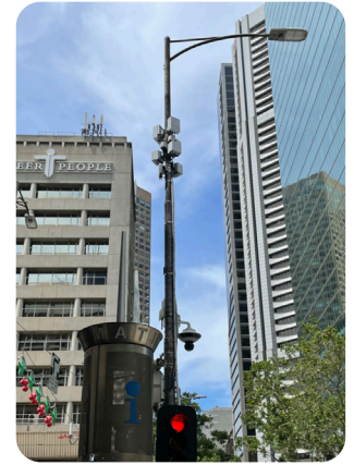
Example 5G small cells installed on street poles
